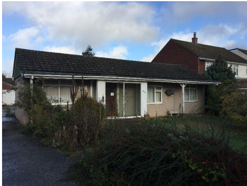
Figure 2: Existing bungalow with garage to rear and No. 38 to side
